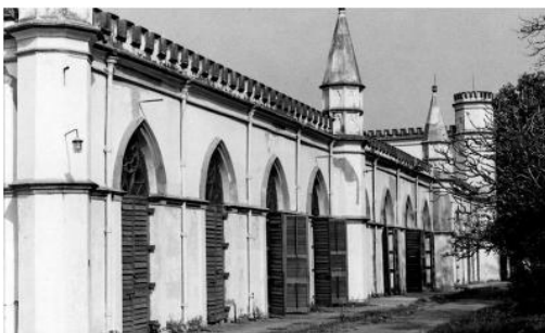
The main workshop complex
